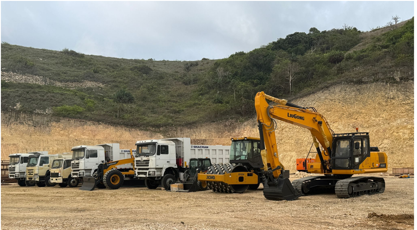
Image 7: Construction fleet expanding with construction works.
