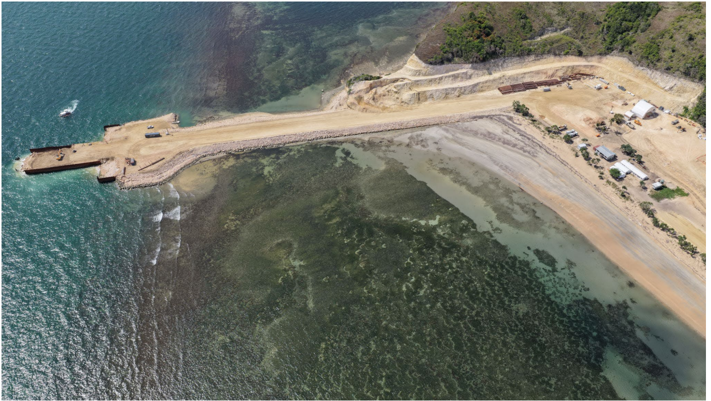
Image 3: Wharf construction is continuing.
