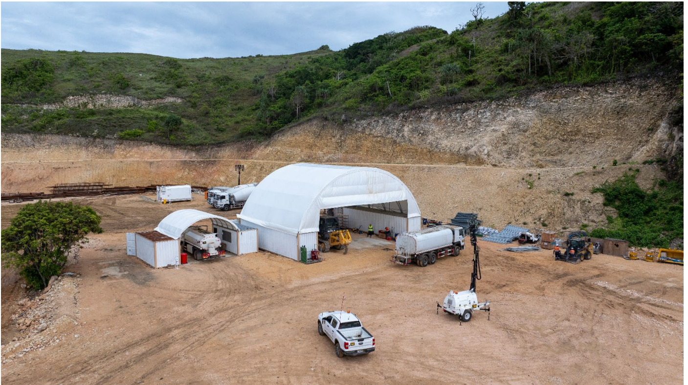
Image 5: Maintenance workshop completed and in use.
