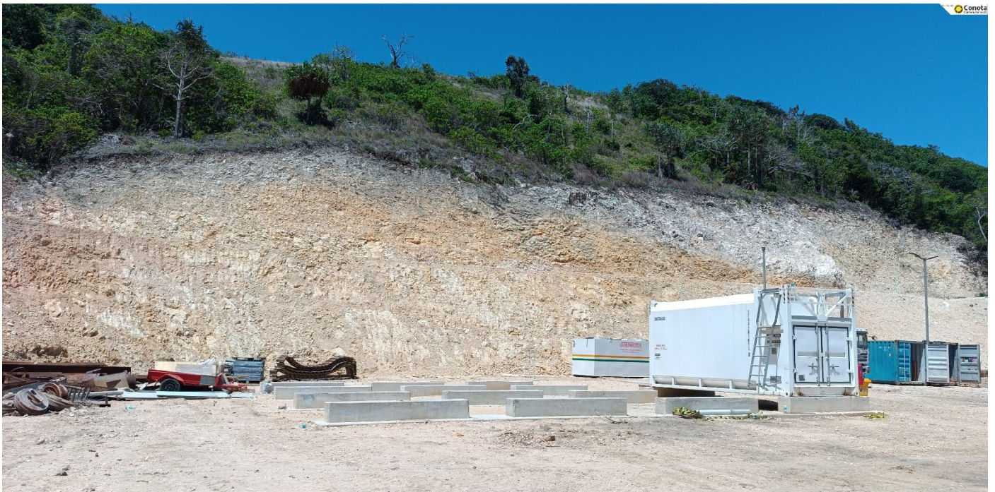
Image 2: Fuel storage foundations have been completed.
