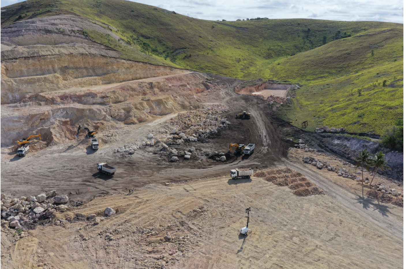
Image 1: Cutting for the kiln foundations are on track for completion.
