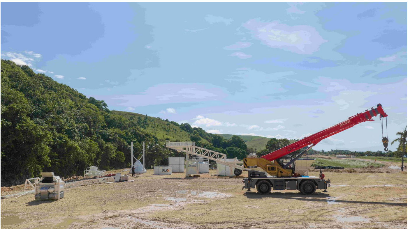
Image 8: Crawler crane and rough terrain crane have arrived.
