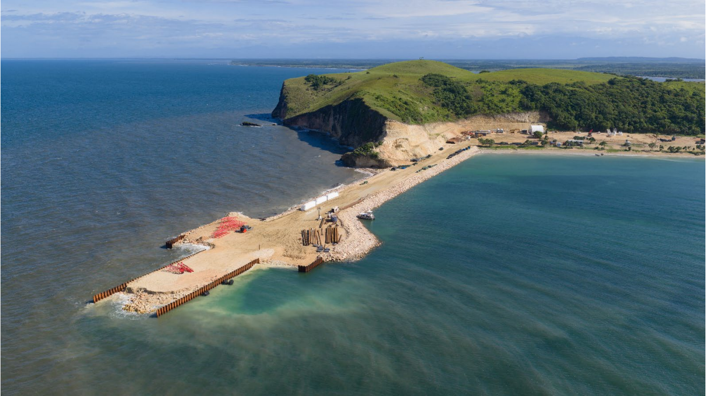
Image 1: Sheet piling for Stage 3 of the wharf is continuing.
