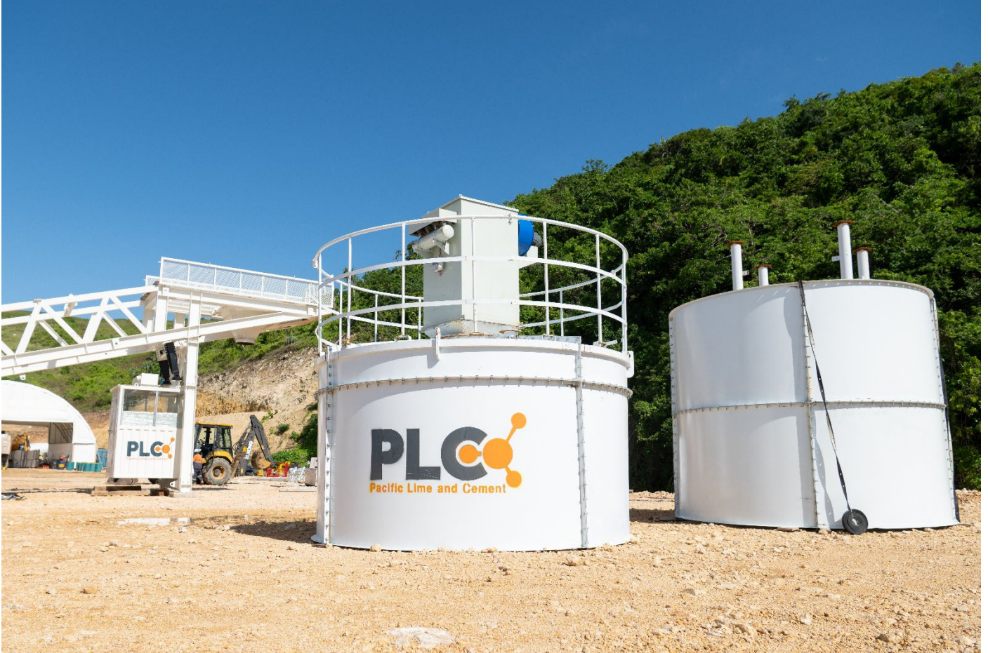
Image 7: Silos and other equipment have arrived at site.
