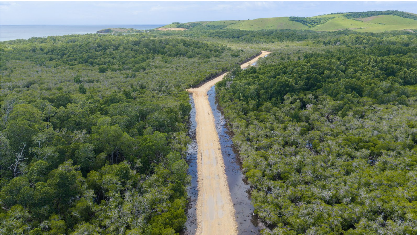
Image 5: Site Access road is progressing well.
