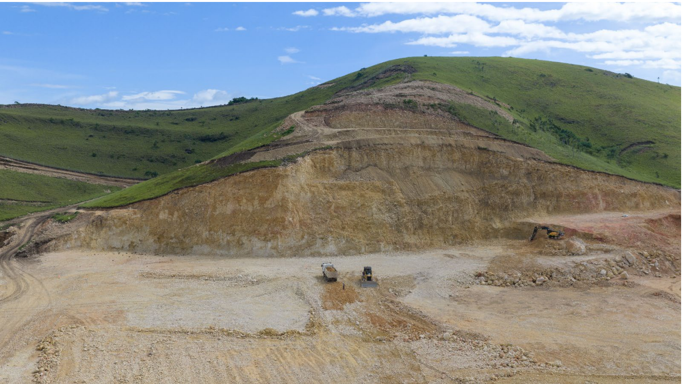
Image 6: Kiln cutting has been blasted down to final level.
