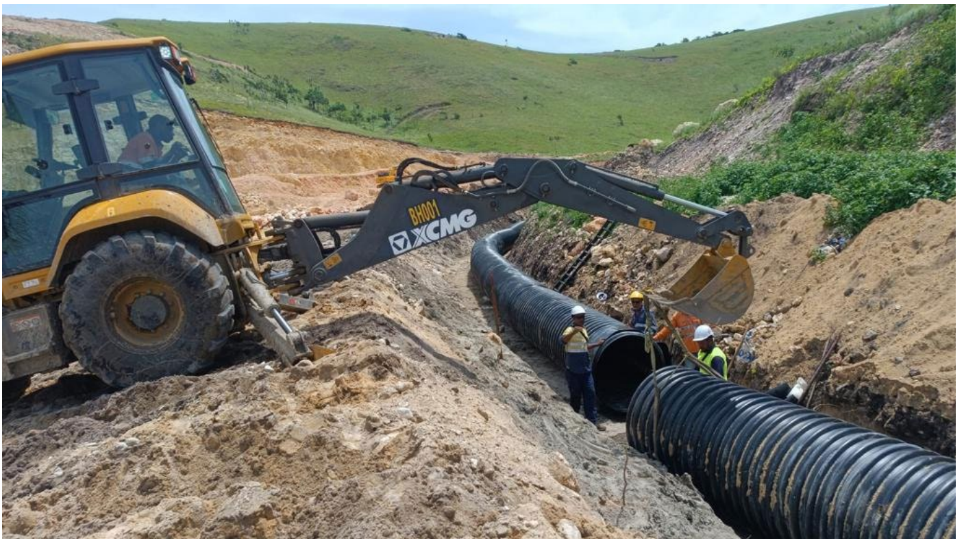
Image 10: Drainage installation pipe and culverts underway.
