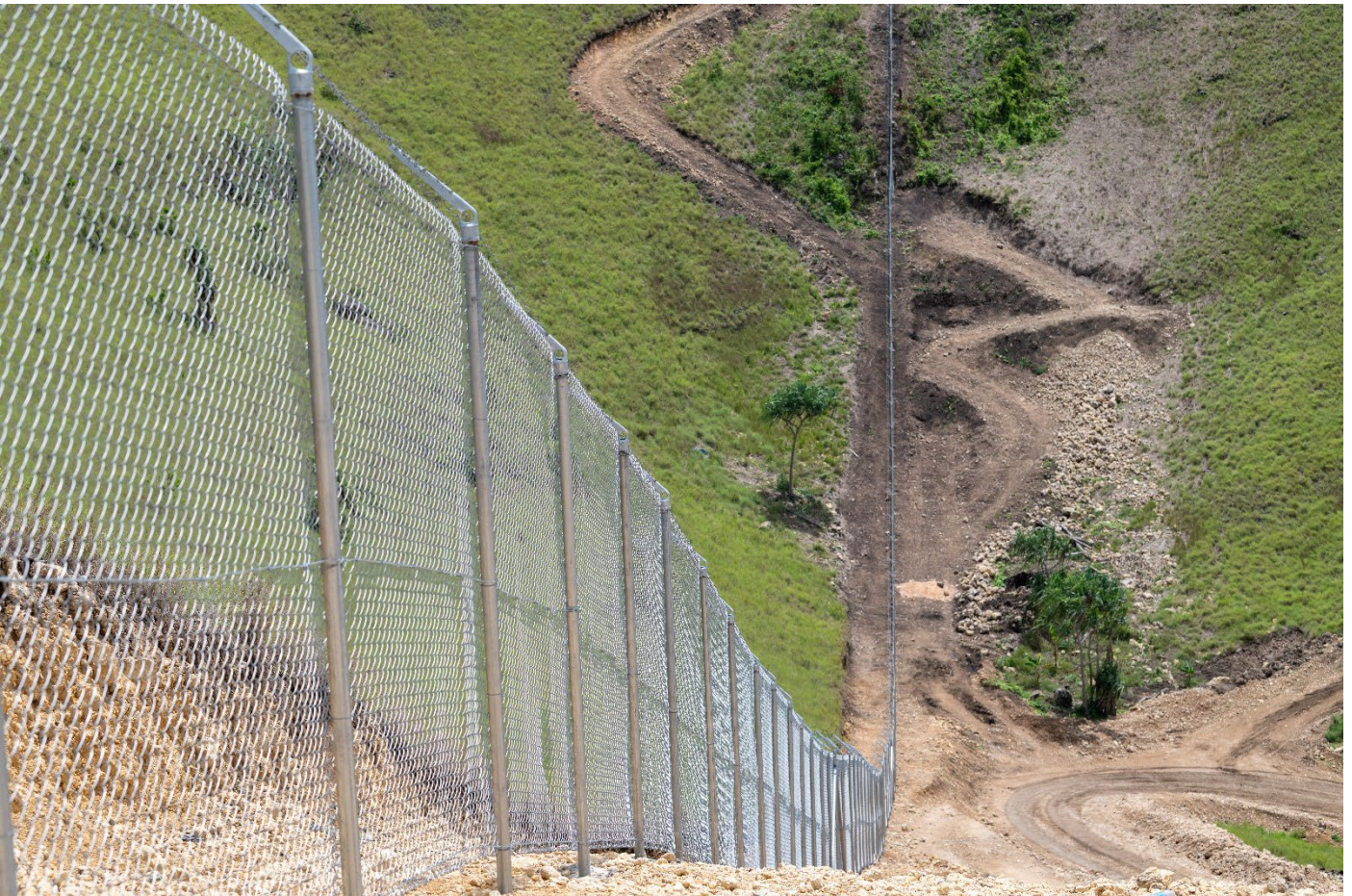
Image 4: Site boundary fence is nearing 50% complete.
