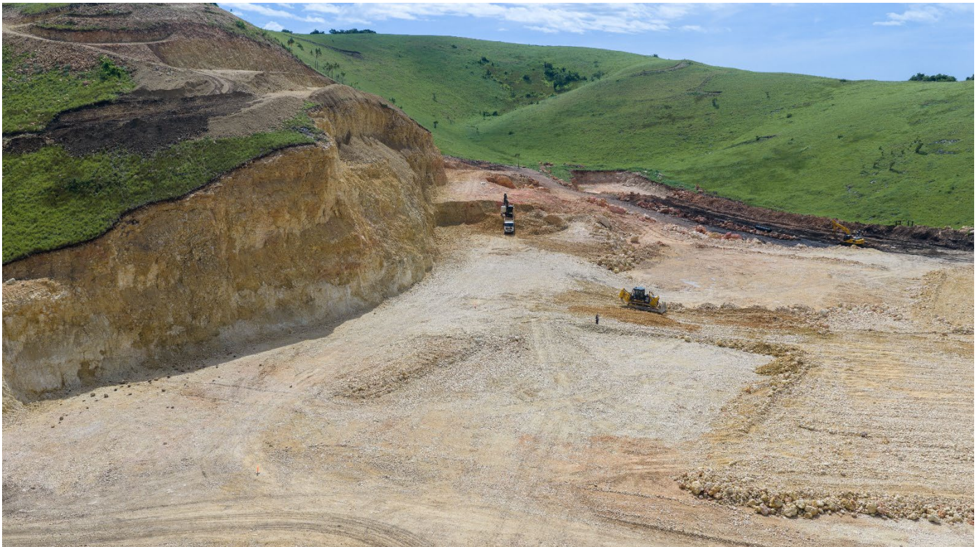
Image: Kiln cutting has been blasted to final level.
