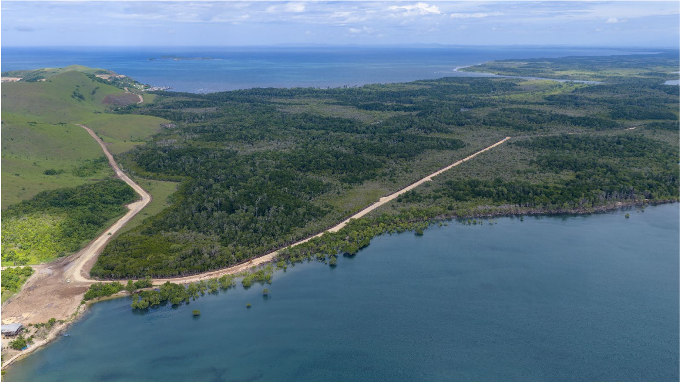
Image: Site access road is progressing well.
