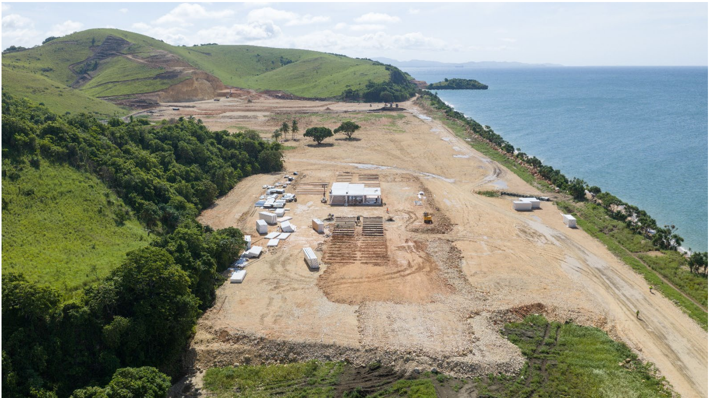
Image: Batch Plant foundations and construction of Camp prefab buildings.
