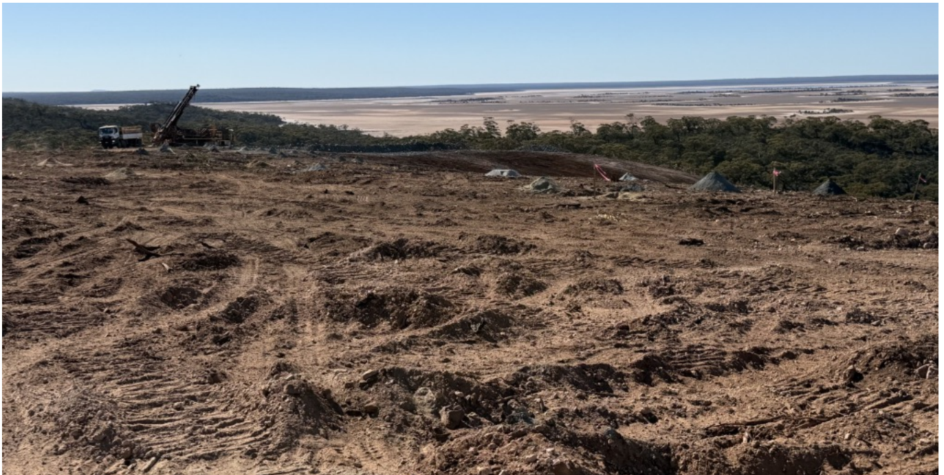
Green Lantern Stage 2 cleared and grubbed with grade control drilling underway.
