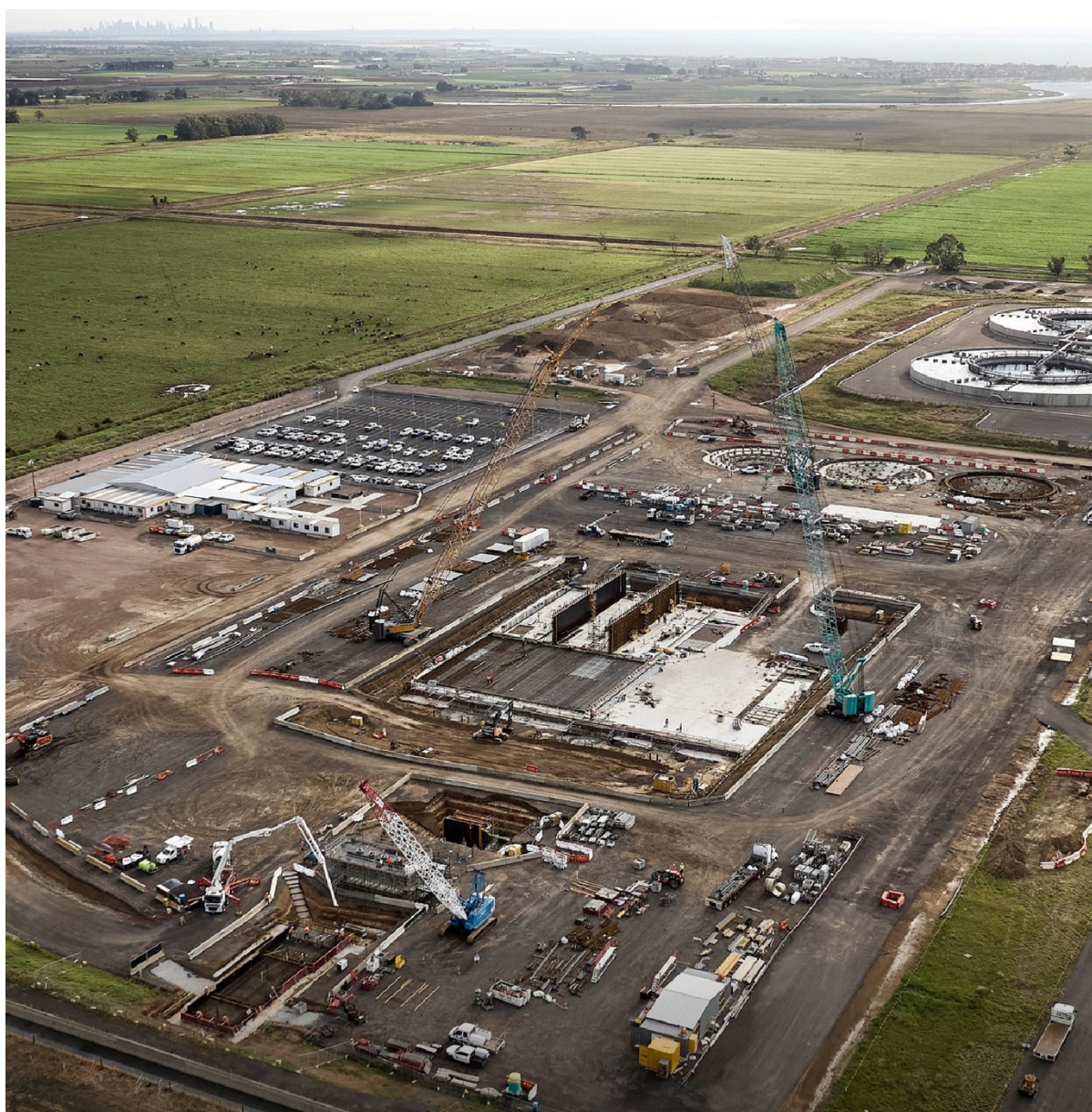
Figure 1: Major Resource Recovery Project – Under Construction
