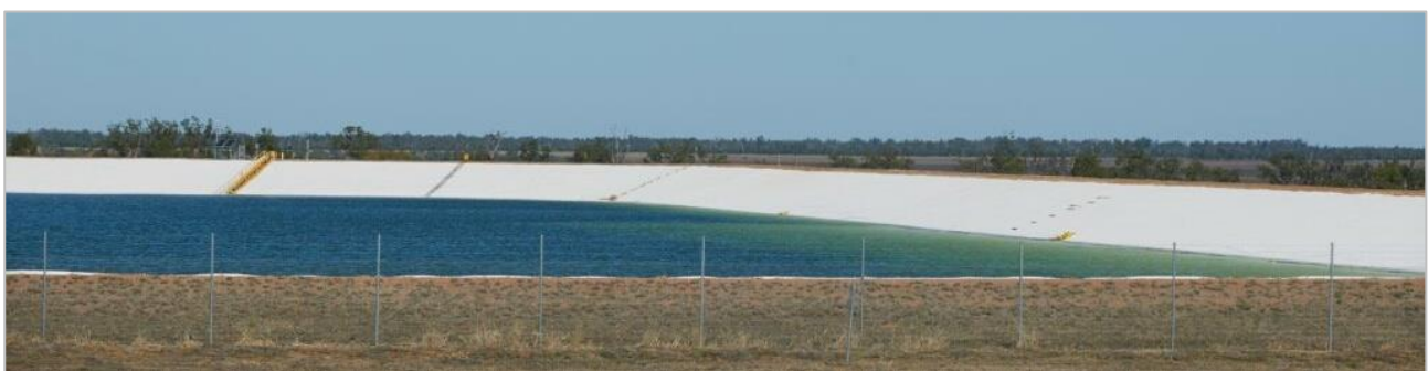
Figure 3.1 CSG brine dam (GISERA, 2026)
