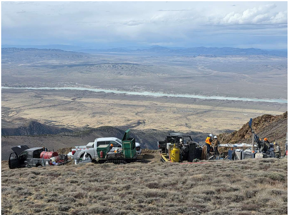
Figure 6. RC rig drilling Ridgeline target, Humboldt Range, Nevada, view west.
