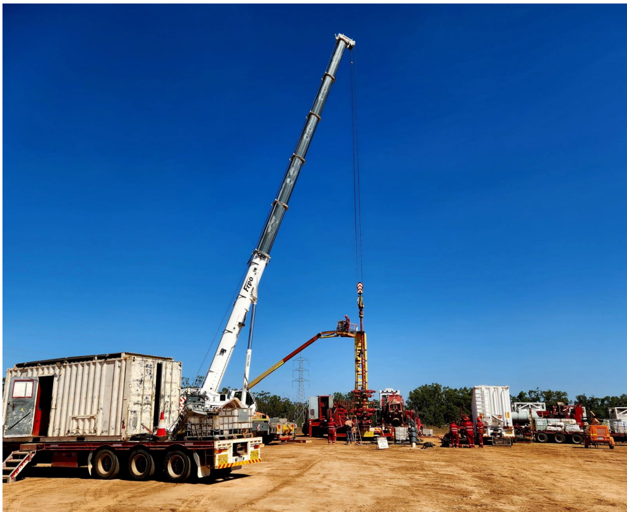
Image: Coil Tubing Unit cleaning out laterals
