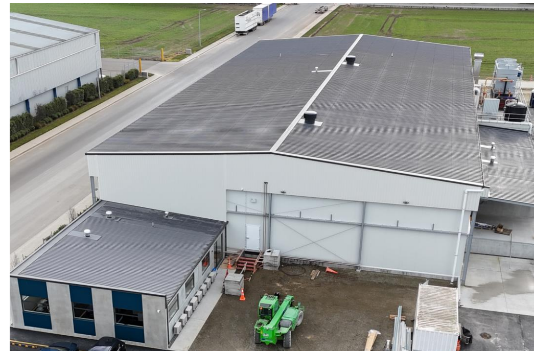
OMP Timaru, South Island, New Zealand: greenfield facility, providing both scale and more efficient plate freezing technology
