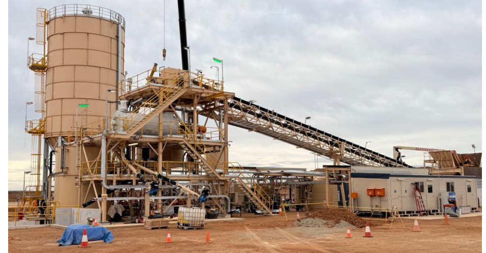
Paste plant nearing commissioning
