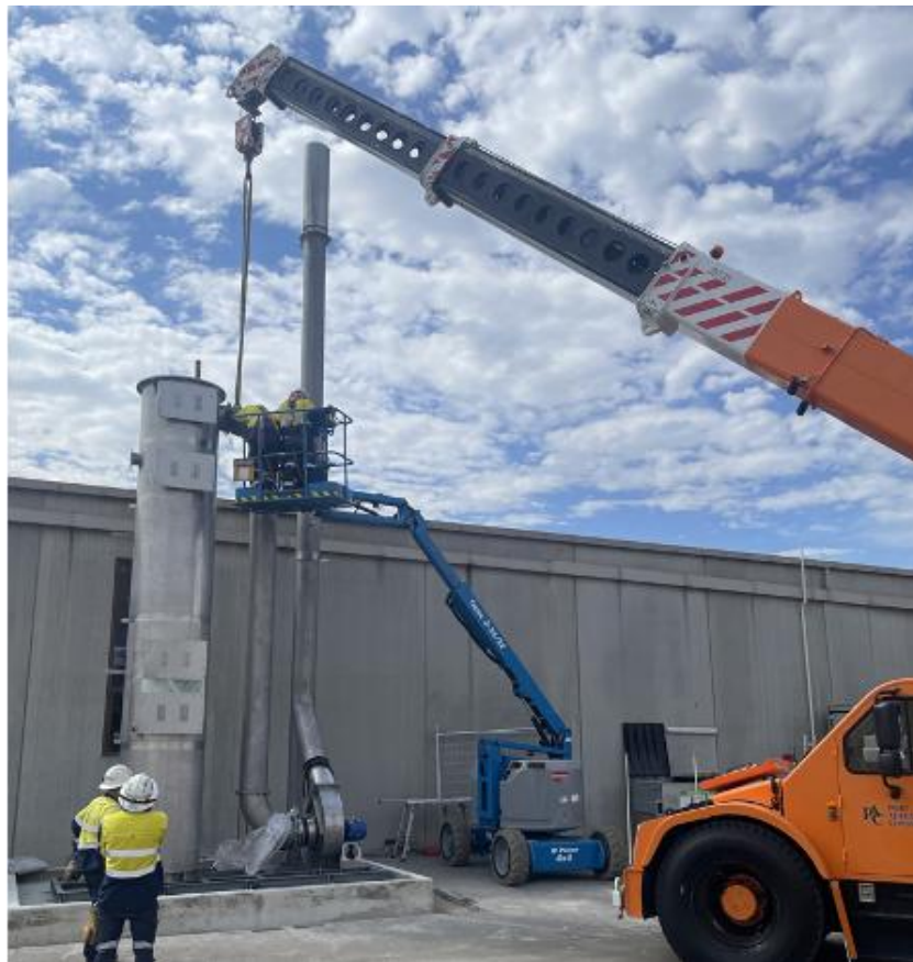
Figure 4. Installation of scrubber at PSG demonstration facility
