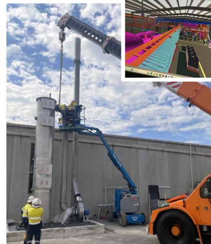
Installation of scrubber
