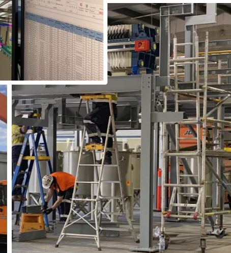
Installation of filter presses
