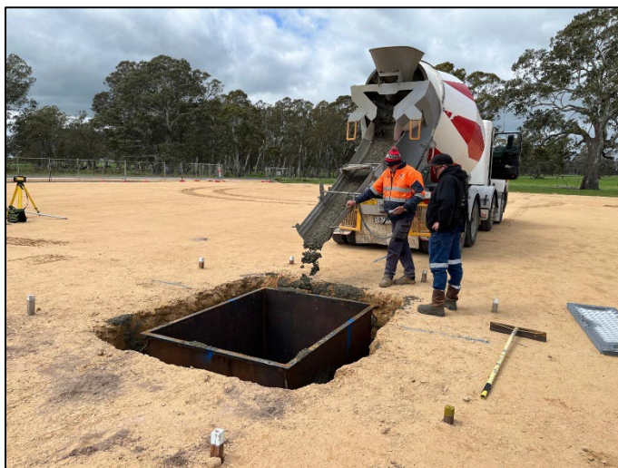
Figure 10 -11: Cellar completed at Killanoola Oil Field (PRL-13)(October 2025)
