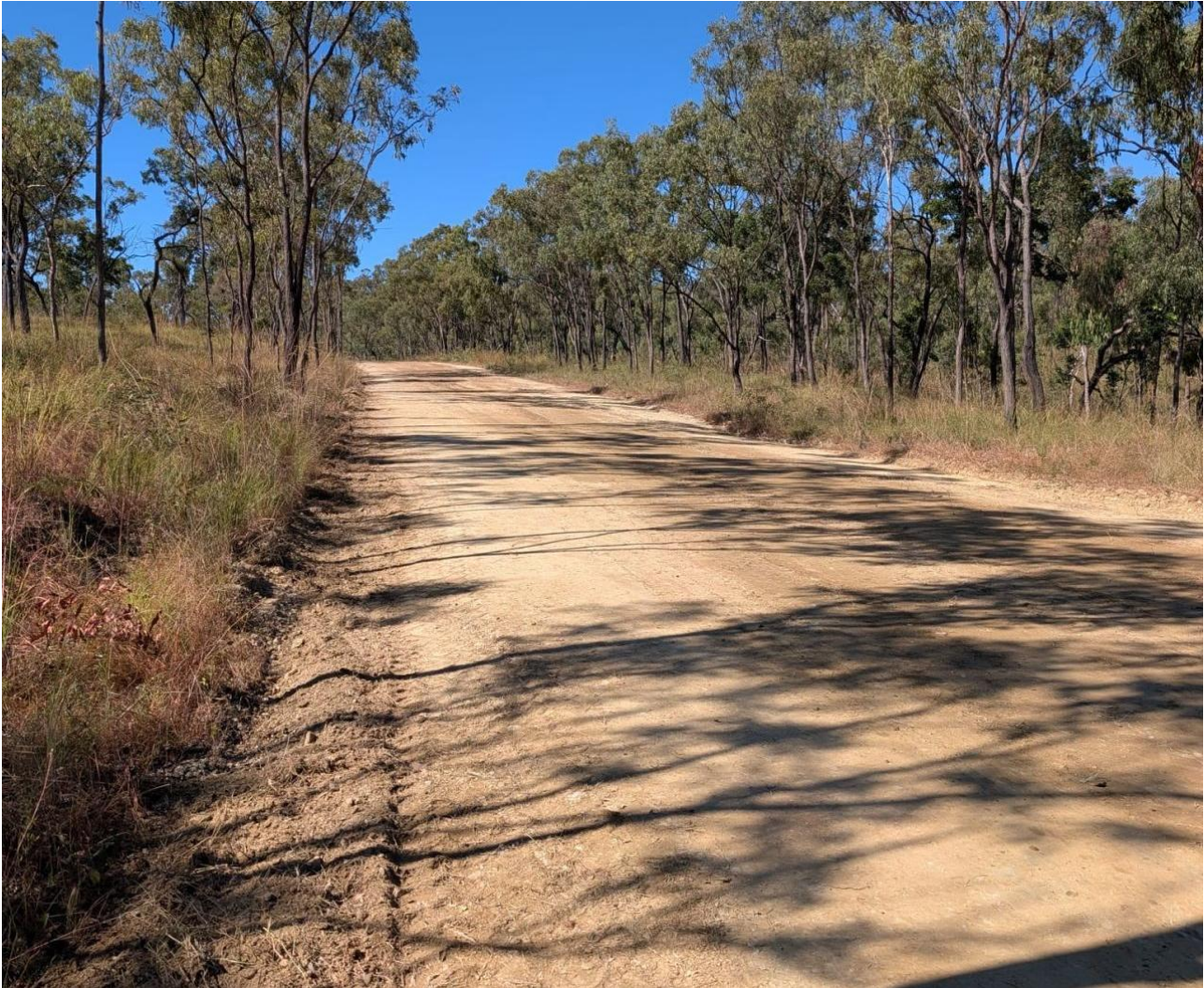
Figure 1: Dianne Copper Mine Project site access road
