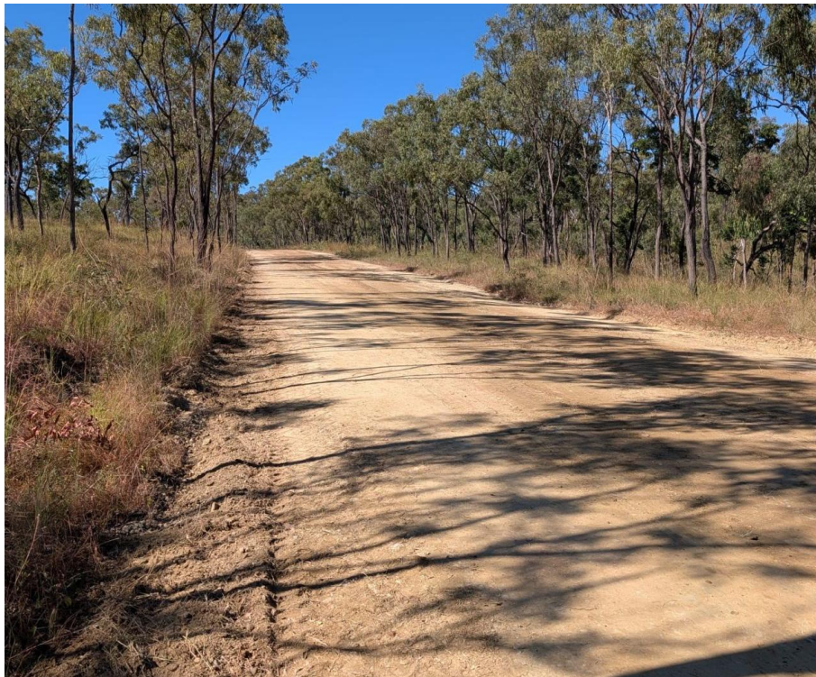
Figure 2: Dianne Copper Mine Project site access road
