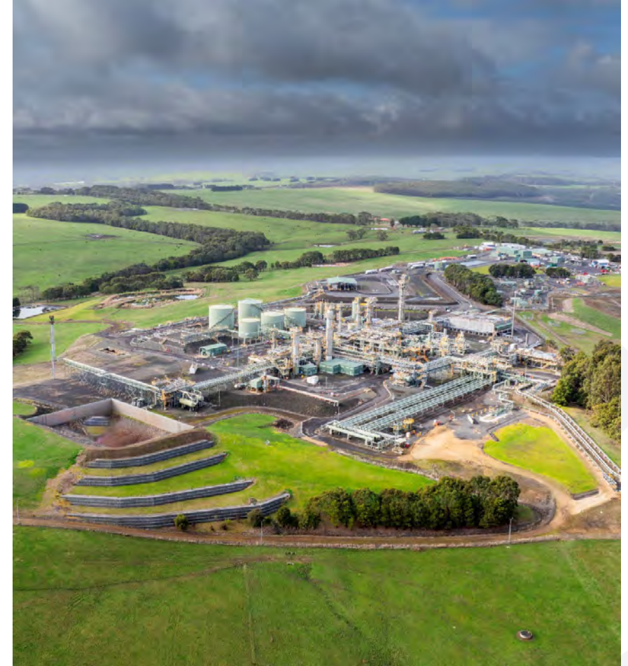
Otway Gas Plant
