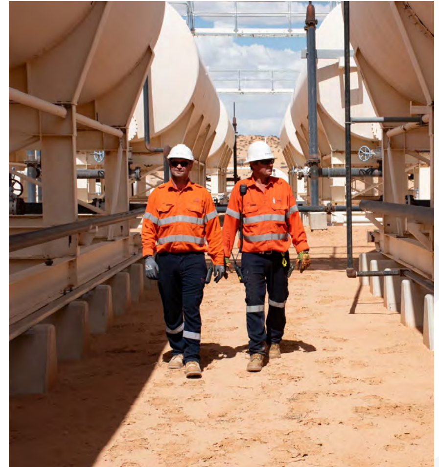
Western Flank, Bauer North Tank Farm
