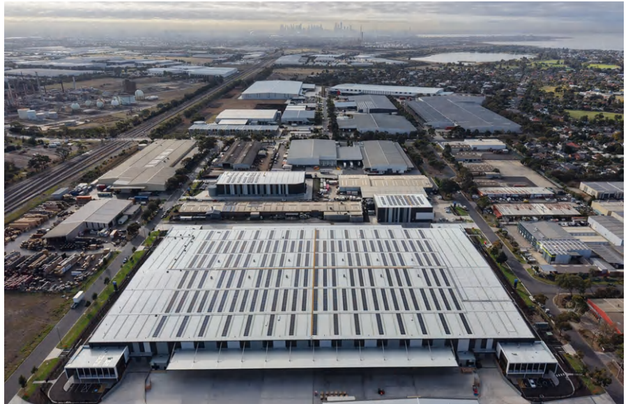
Energy Bay solar at Altona Distribution Centre, Vic
