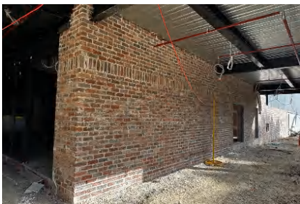
Reused bricks at Yennora Distribution Centre, NSW
