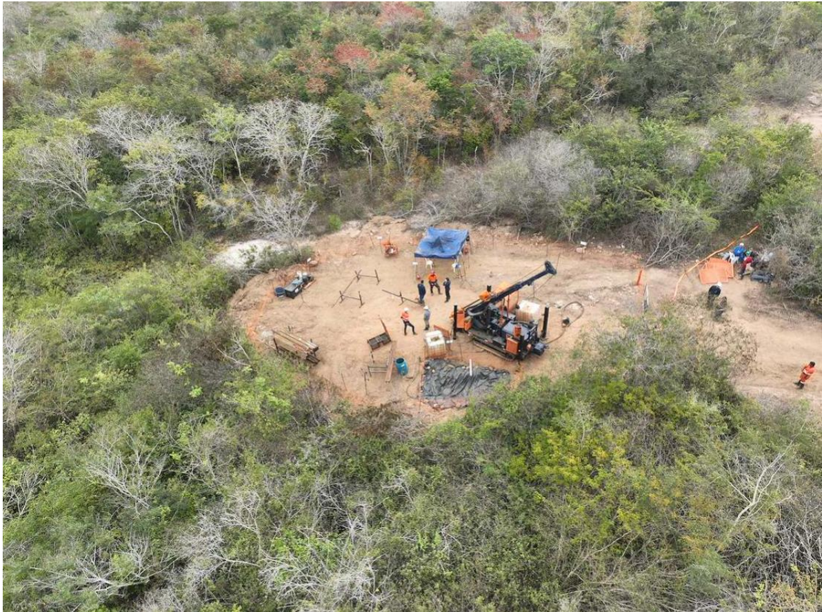
Figure 5: drill rig mobilised at Mandacaru (pad reference F-01 (Figure 4)).
