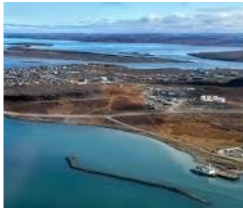
Kugluktuk: Port facility
