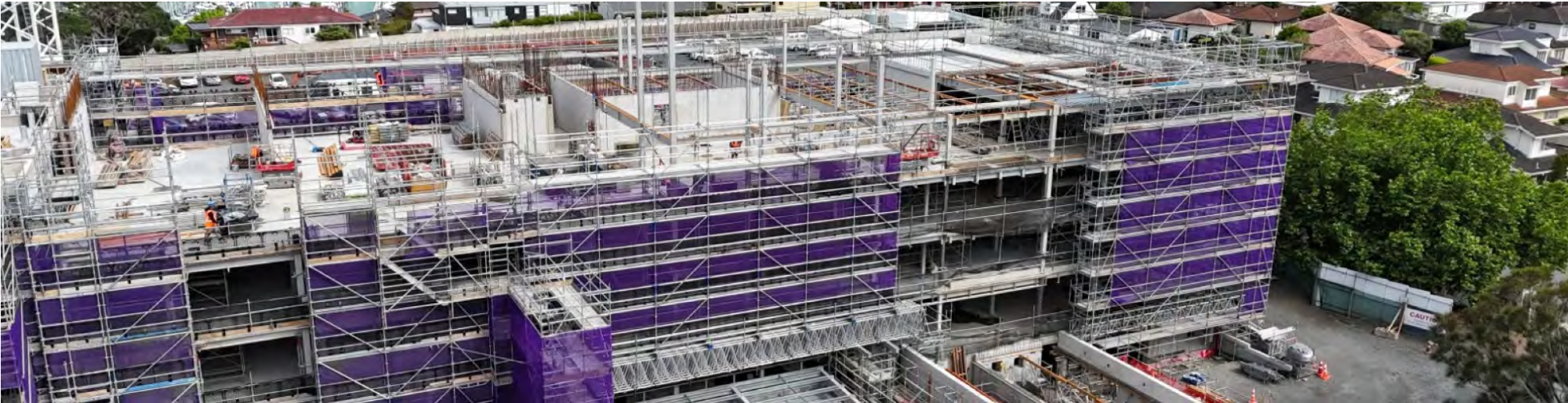
📷 Vertical construction and waste-management in action at Summerset Half Moon Bay
