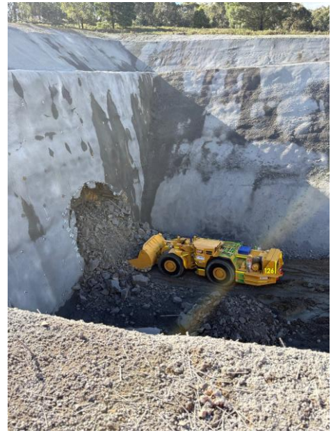
Figure 2. Bogging the first cut from the decline portal.
