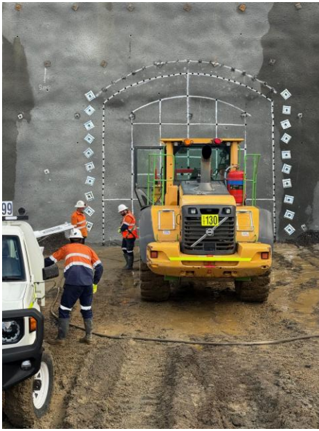
Figure 1. Exploration decline portal, face markup prior to firing.
