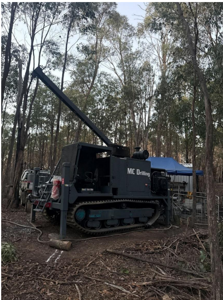
Figure 1: Regional drill rig set up at Redcastle.
