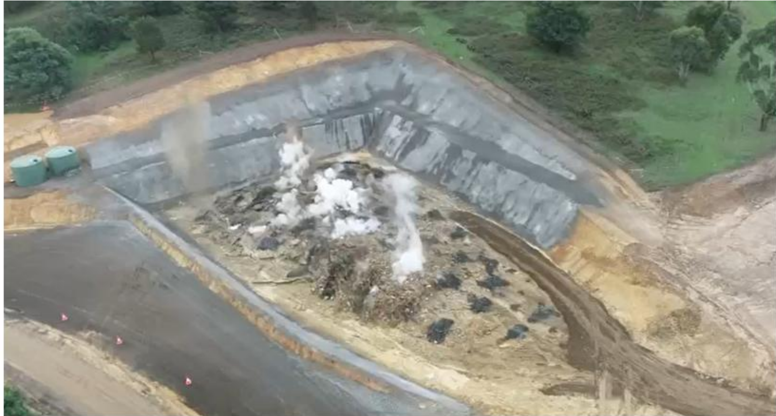
Box cut blasting
