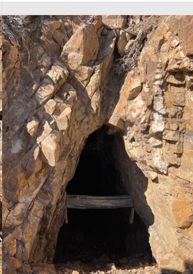
Figure 3: Northern adit entrance
