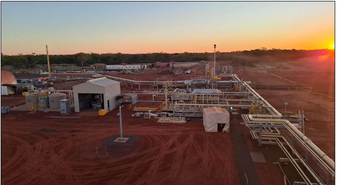
Figure 2: Construction activities of the SPCF
