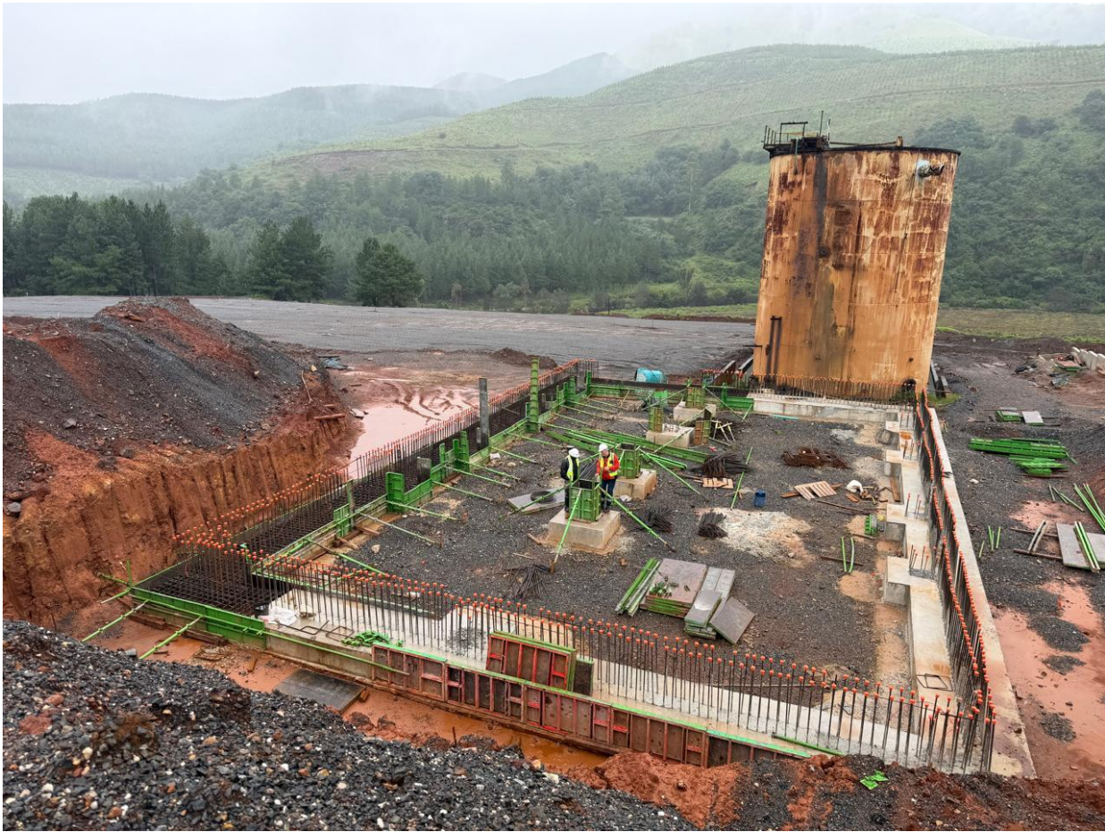
Figure 2: Civil works underway for Gold Room foundations.
