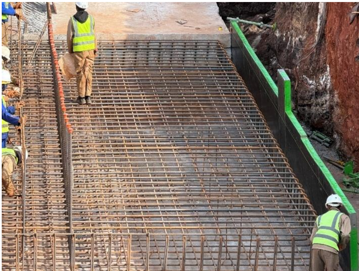
Figure 4: Retaining wall foundation steelworks
