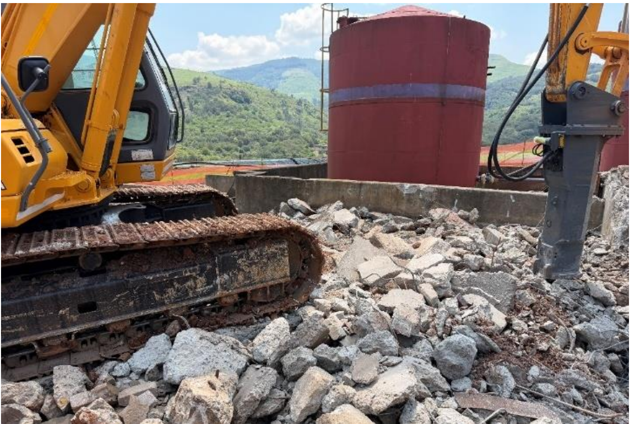
Figure 3: Removing old engineering structures
