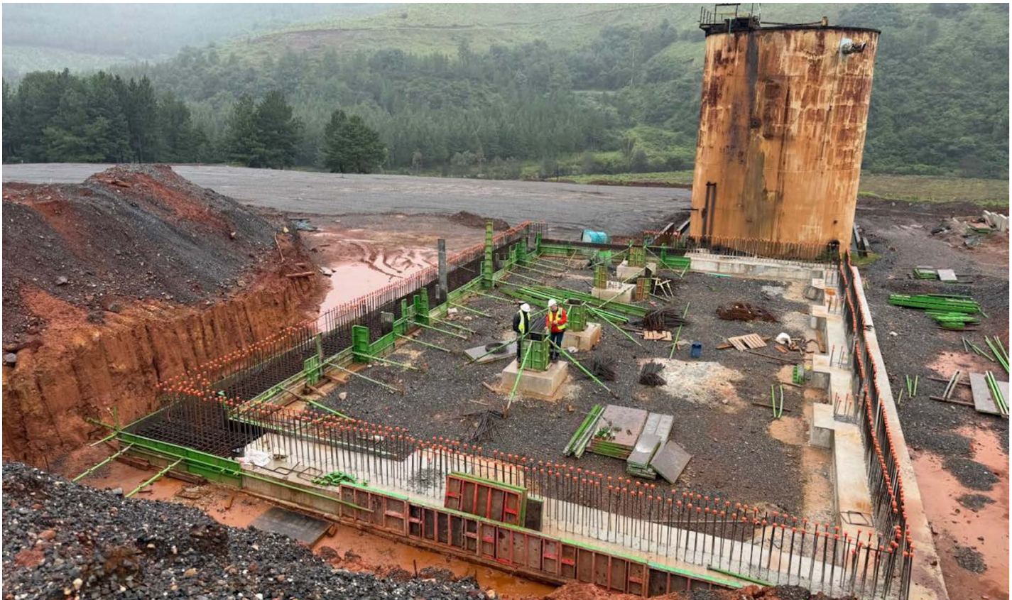
Figure 3: The Gold Room's Foundations
