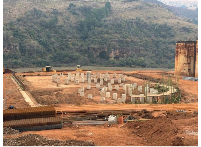
Figure 5: Thickener tank/processing area foundations
