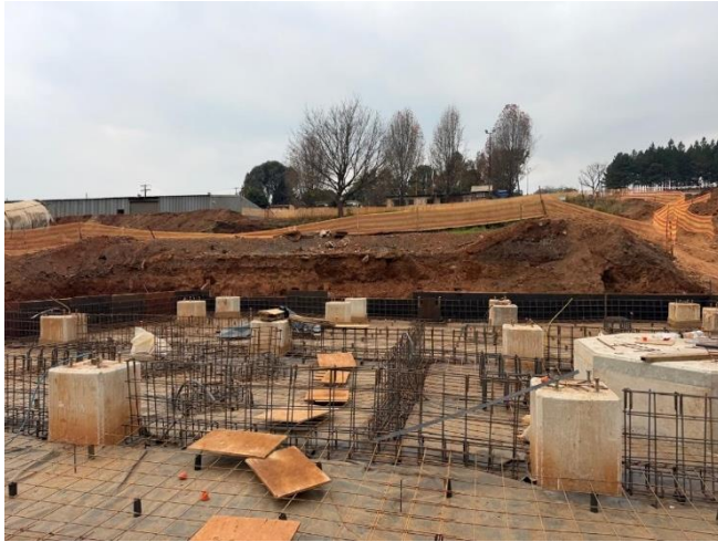
Figure 4: Elution circuit foundations
