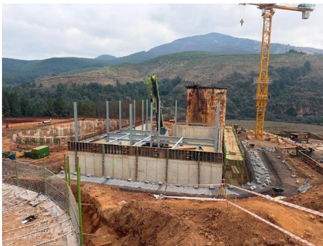
Figure 6: Gold Room construction continues - steel works
