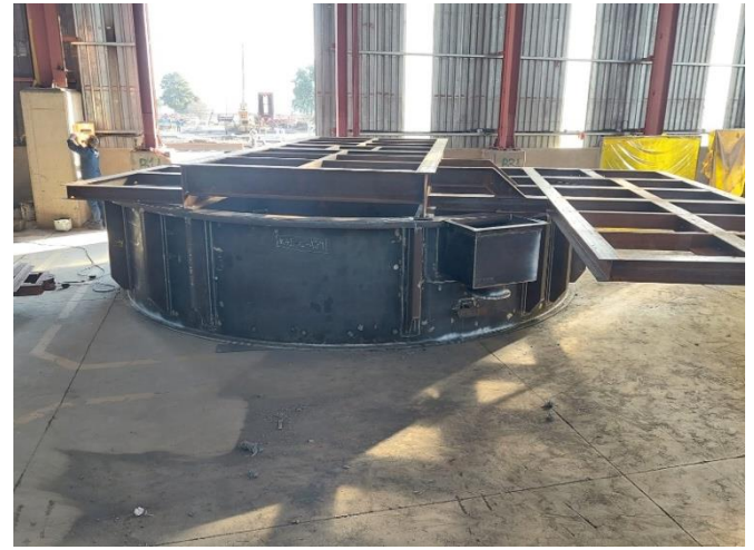
Figure 7: CIL Tank fabrication
