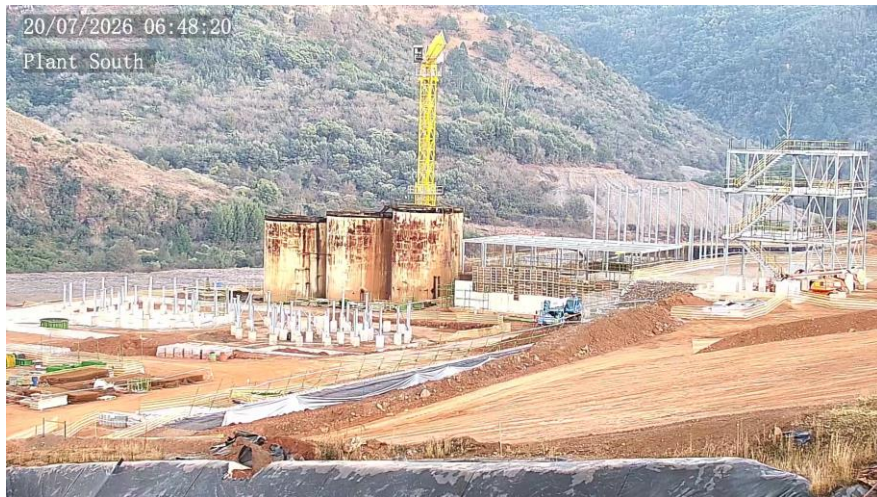
Figure 14: South view of the plant – indicating the civils for the crushing and screening plant
