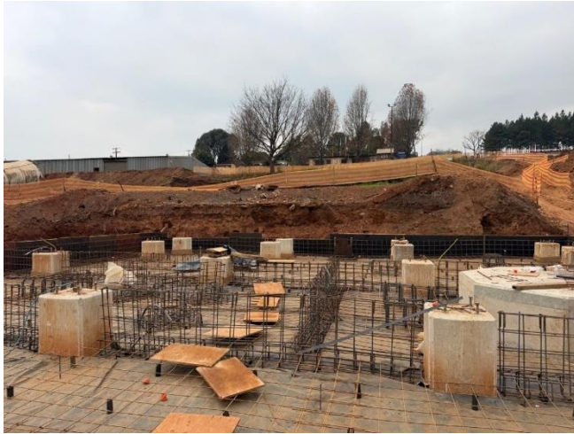
Figure 6: Elution circuit foundations
