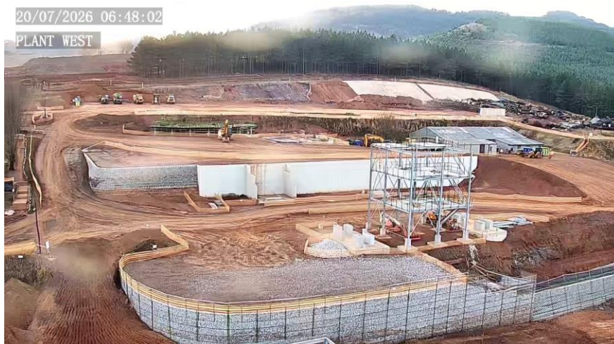
Figure 13: West view of the plant – indicating the gold room and elution buildings
