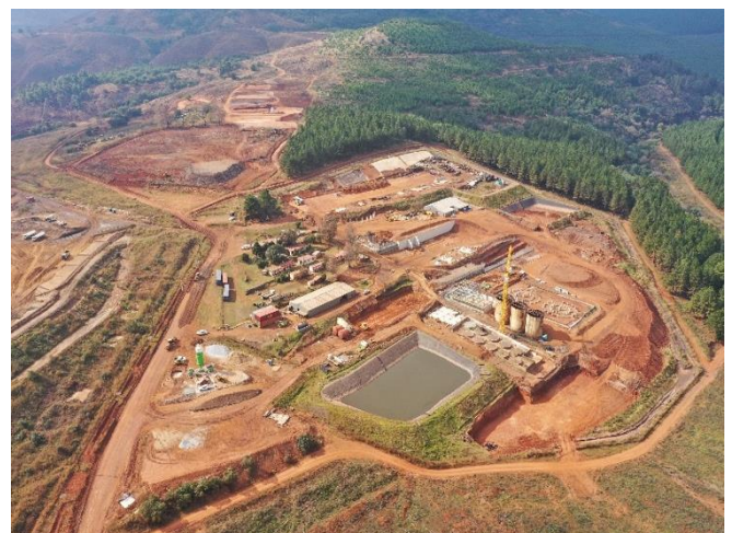
Figure 5: Site aerial view highlighting plant footprint and integrated construction progress
