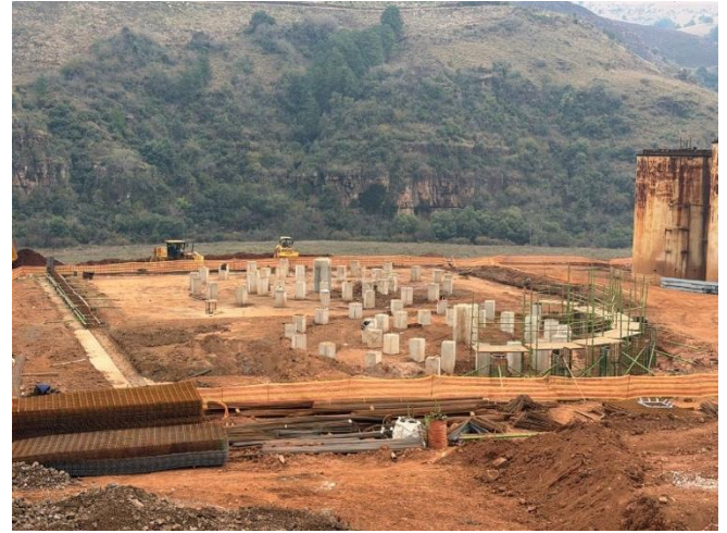
Figure 7: Thickener tank/processing area foundations
