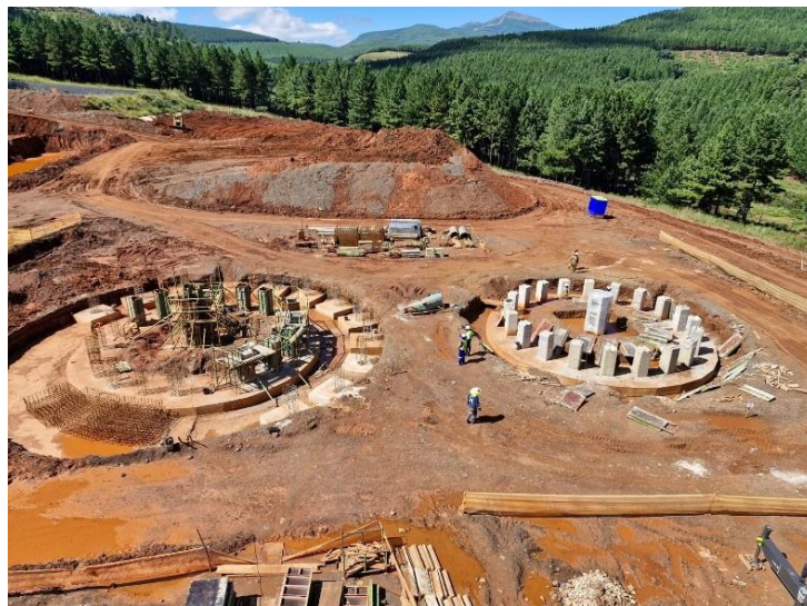
Figure 12: Thickener Tank foundations in progress
