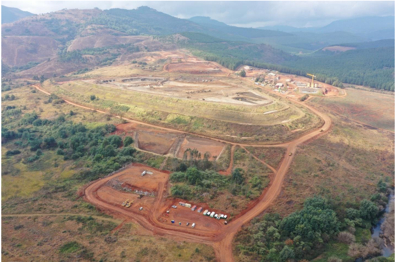
Figure 3: TGME Gold Project aerial view of the TSF (bottom: Laydown area ; middle: TSF; top right: new plant under construction).
