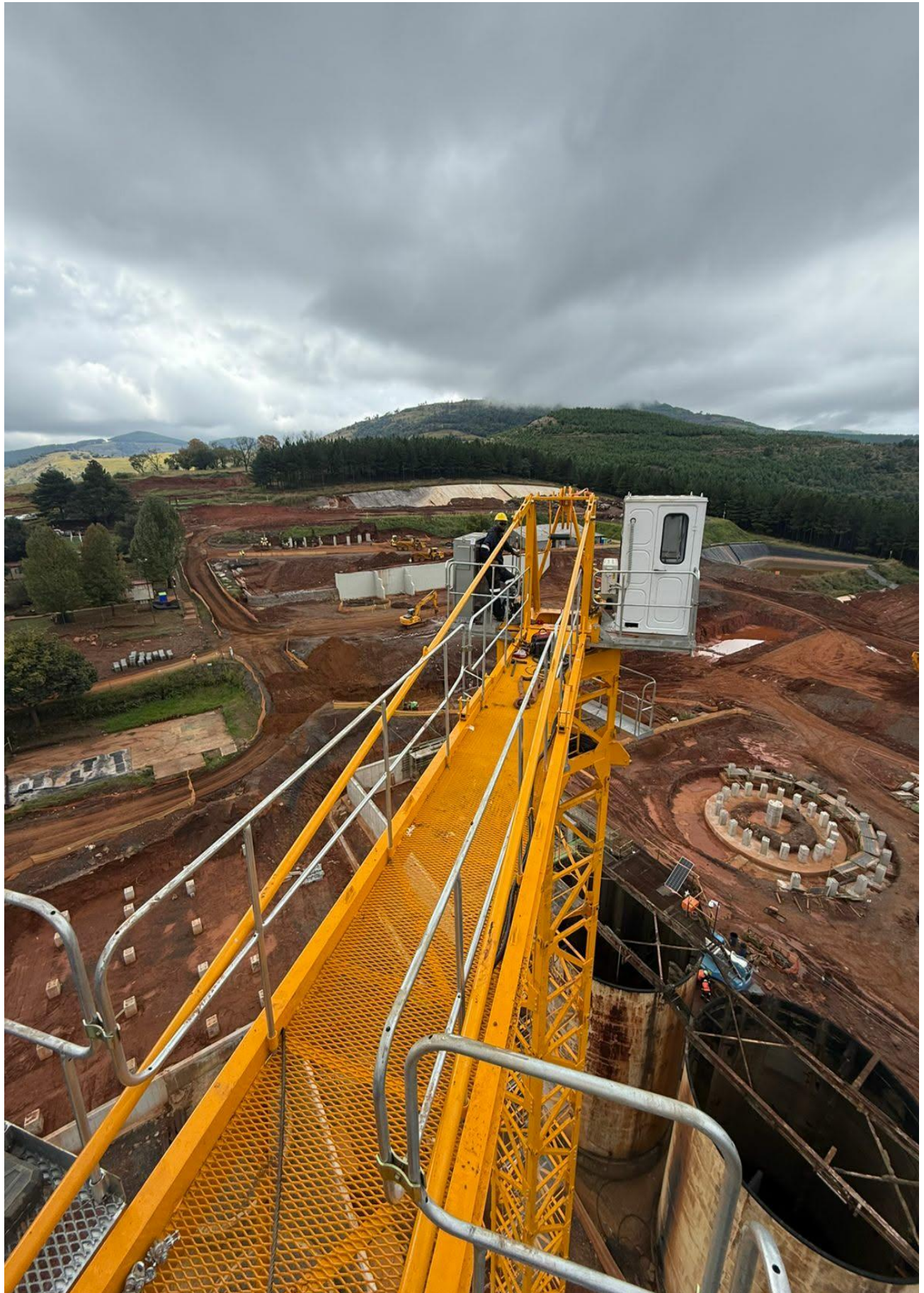
Figure 18: Stationary Crane now fixed in place at site for construction and maintenance
