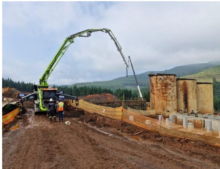
Figure 11: Concrete Pumping – Gold Room
