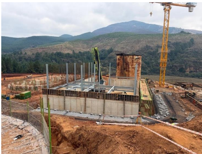
Figure 8: Gold Room construction continues - steel works
