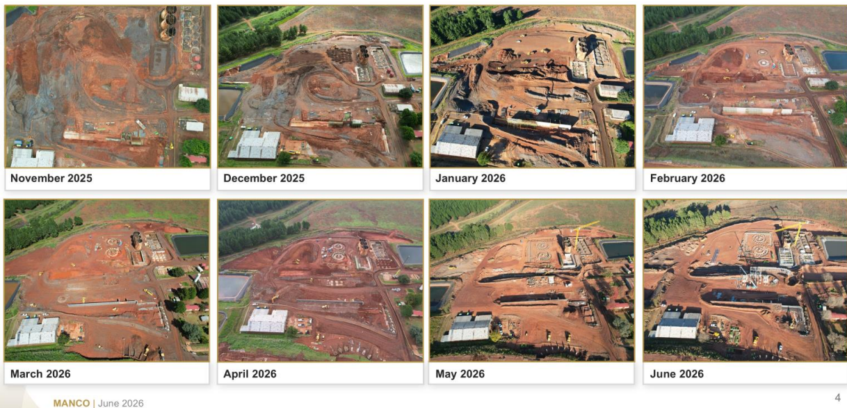
Figure 2: TGME Gold Project – Time Lapse Construction Photos
