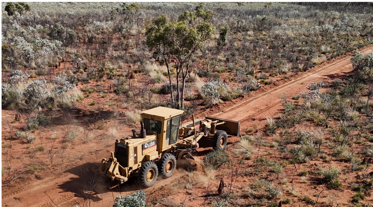
Figure 1. Pre-drill earthworks have commenced at regional drill targets under the supervision of Jaru monitors.
