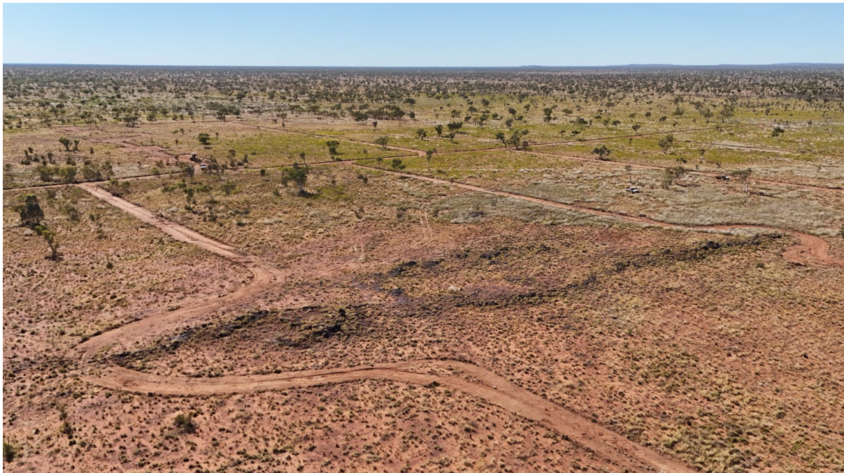
Figure 1. Pre-drill earthworks have commenced at Kuro under the supervision of Traditional Owner monitors. Drone photo above showing drill tracks and the prominent black discovery outcrop.
