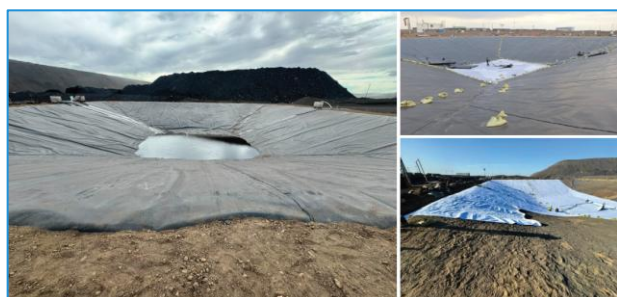
Figure 3 – Pond maintenance completed.
