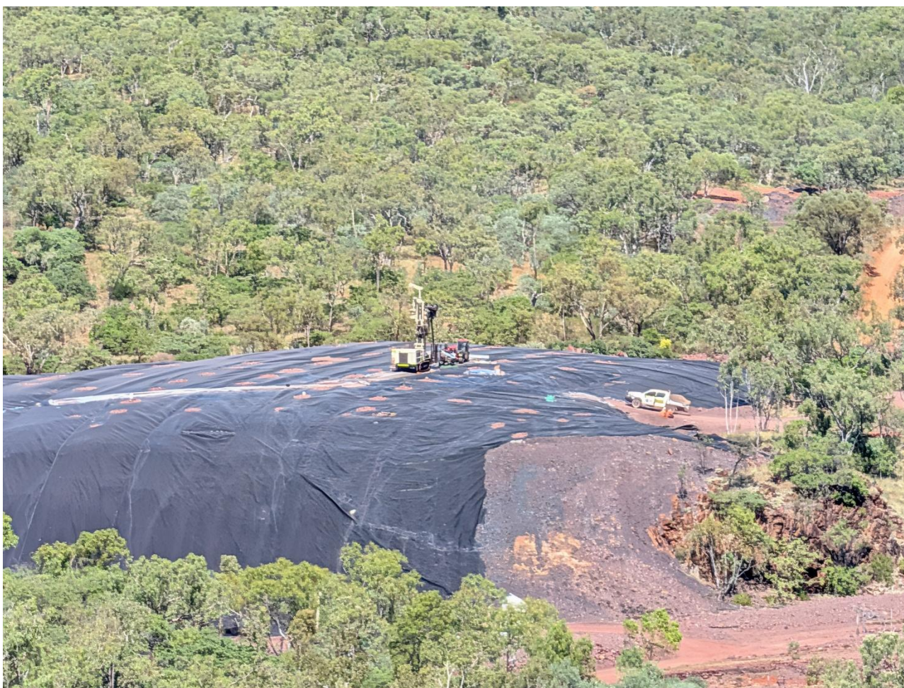
Figure 6 . Sonic drilling rig conducting a characterisation drill program on a legacy mine materials stockpile at Mount Oxide.
