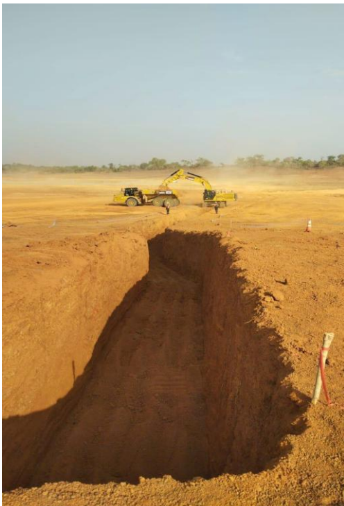
Figure 5: Excavation of embankment of water storage dam
