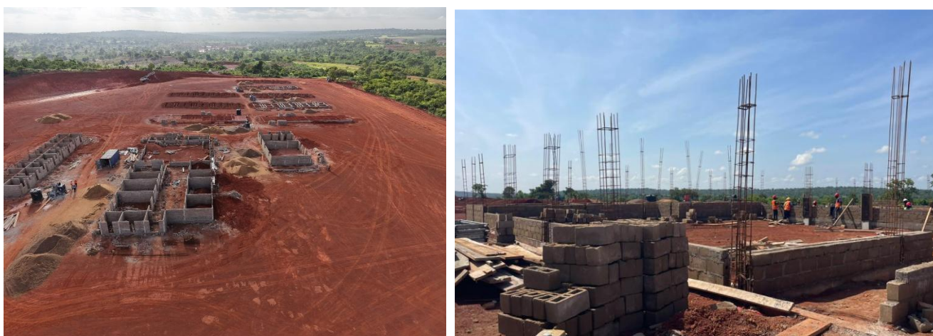
Photos 5 & 6: Construction of accommodation camp
