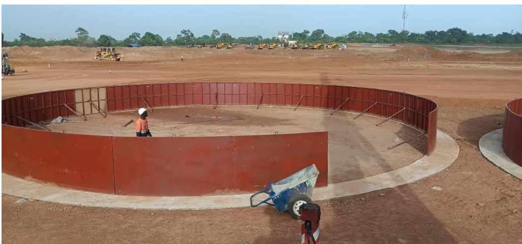
Photo 1 & 2: Process Plant Area at the Kobada Gold Project CIL Tanks - ring beam construction commenced with setting up of formwork
