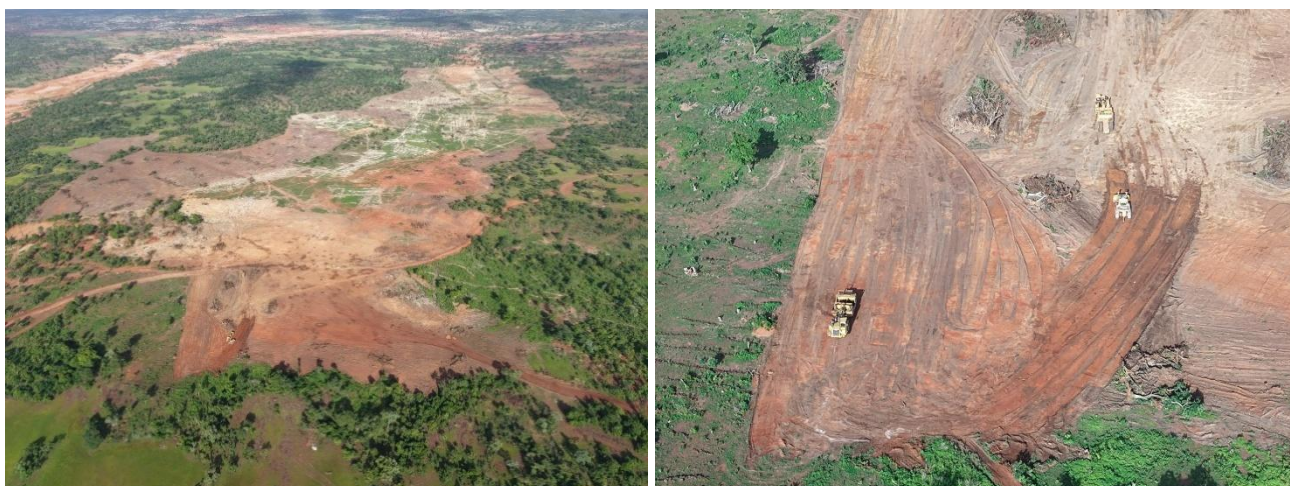
Photos 3 & 4: Clearing of land for tailings storage facility (LHS) and construction of TSF embankment (RHS)
