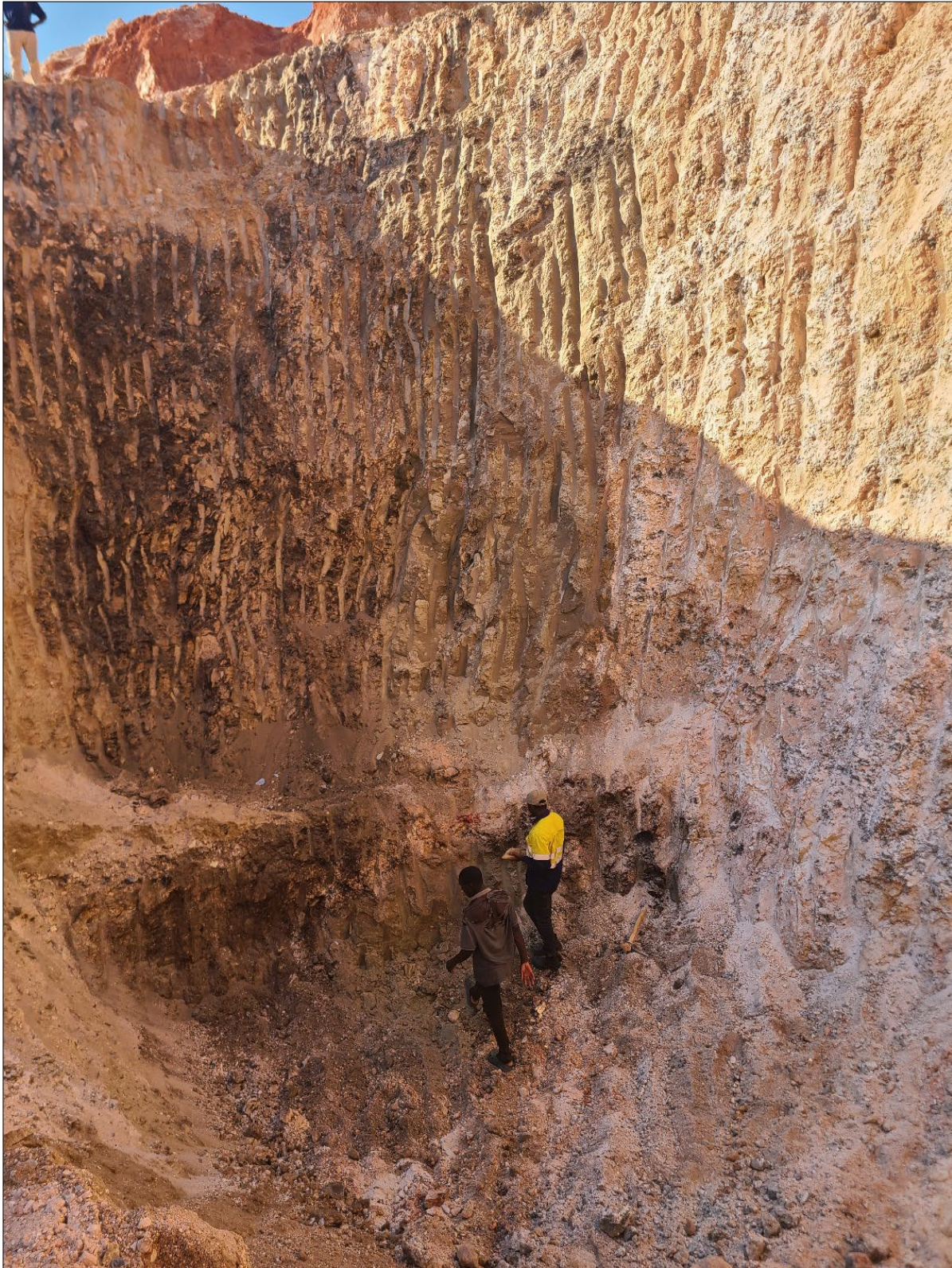
Figure 3: Exposure of a road reclamation pit sidewall showing a well-developed residual weathering profile comprising ferruginous pedolith, mottled clay and saprolitic material.
