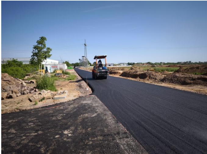
Figure 9: Road resurfacing post ICPP crossing work completion.
