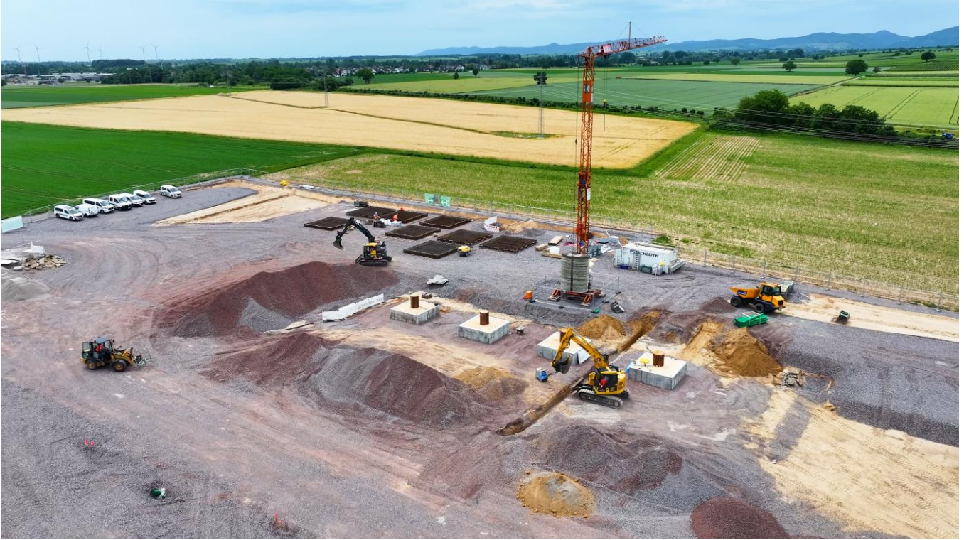
Figure 5: Construction works at the fourth well-site ahead of mobilisation of the second Vercana rig, known as V10, in H2 2026. Poured concrete for all four drilling cellars can be seen in the middle of the image.
