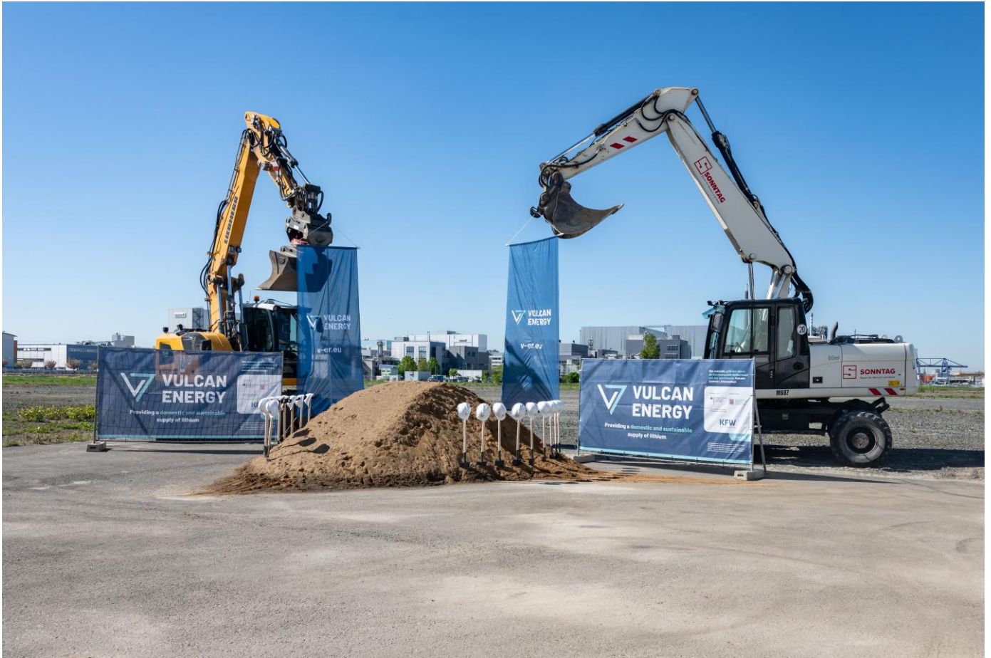
Figure 15: Vulcan held its groundbreaking event for its lithium chemicals plant in Frankfurt in April 2026.
