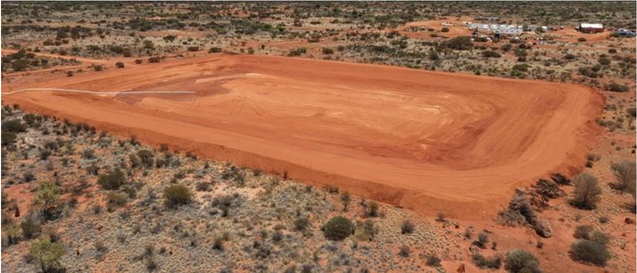
Figure 7: Water-containment sump prepared for the commencement of long-term pump testing
