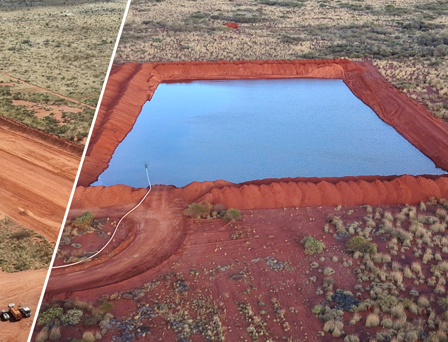
Water sump for long-term pump testing to inform hydrogeological activities
