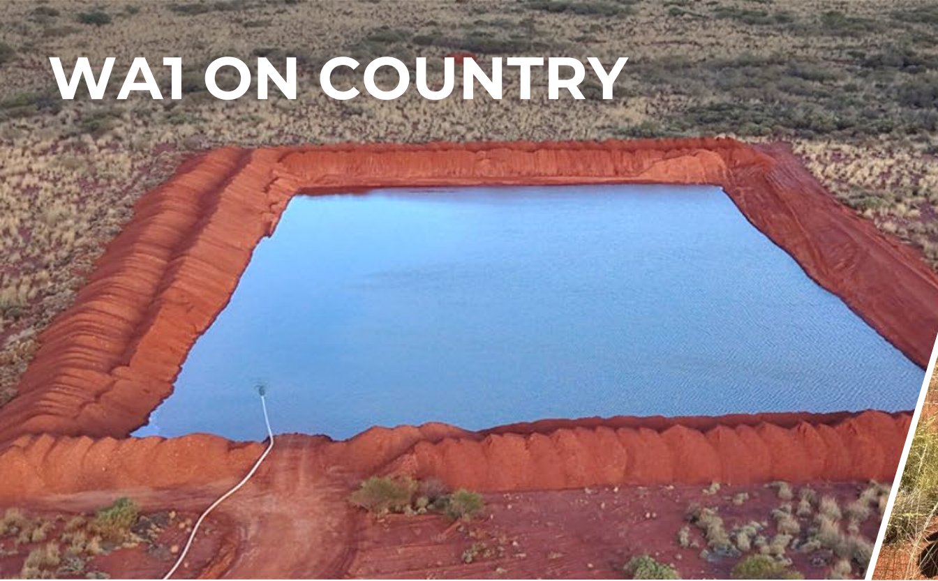
WATER SUMP FOR LONG-TERM PUMP TESTING TO INFORM HYDROGEOLOGICAL ACTIVITIES
