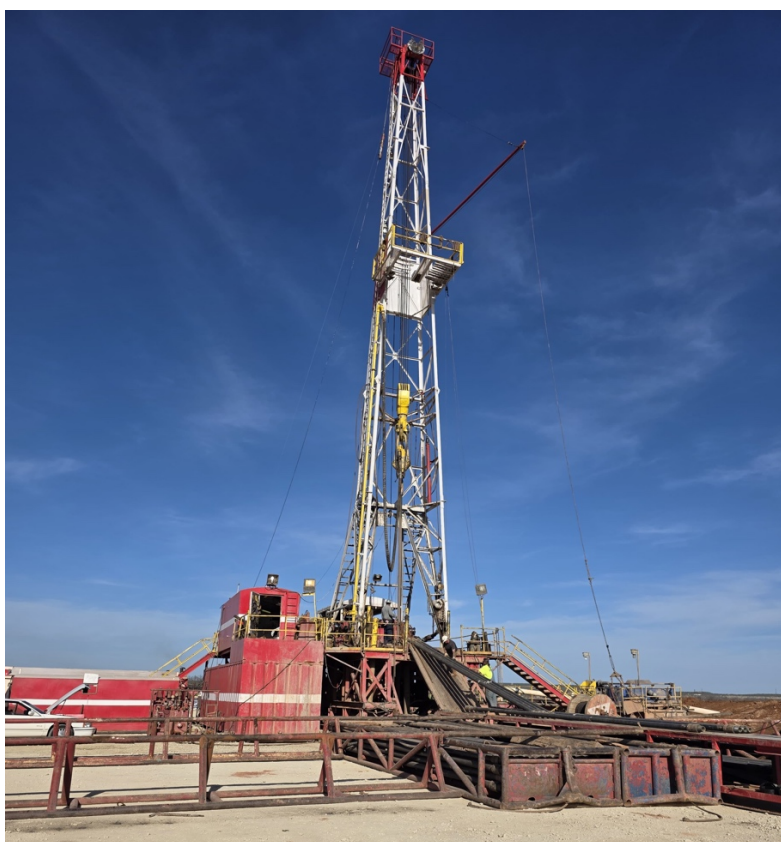
Photo 1: Drilling of the JVU-4 injection well at the Varn Oil Field
