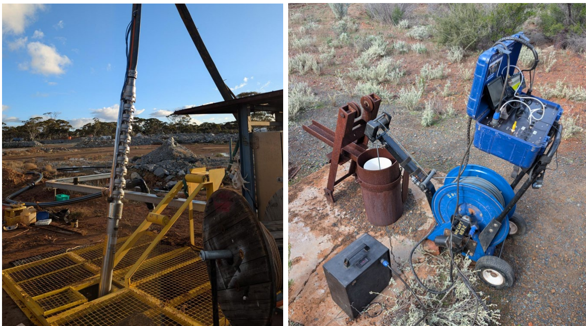
Photo 6 and 7: Dewatering pump being lowered into the shaft and Bore field investigations
