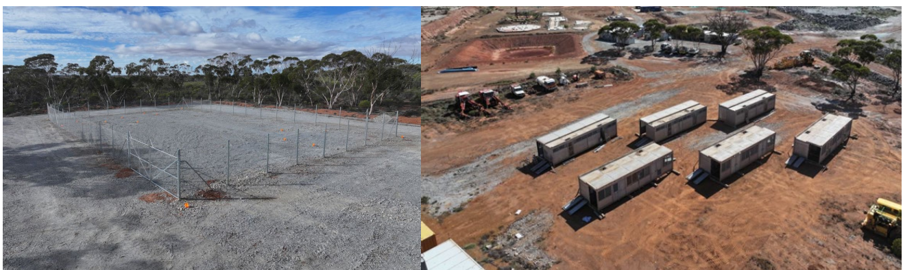
Photo 4 and 5: New magazine fencing and earthing and Widgie dongas undergoing refurbishment
