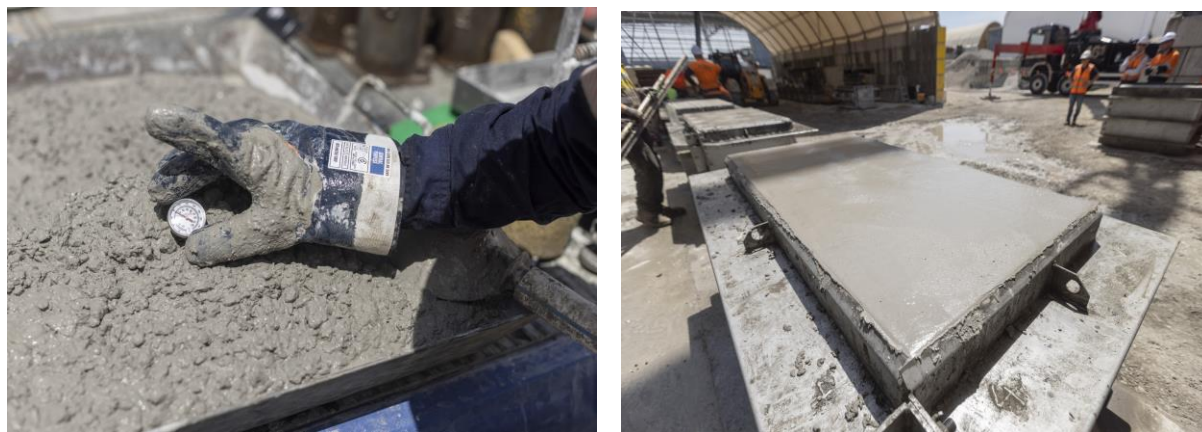
Figure 1 & 2: Wind farm concrete trials - 50% AusPozz™ mix design
