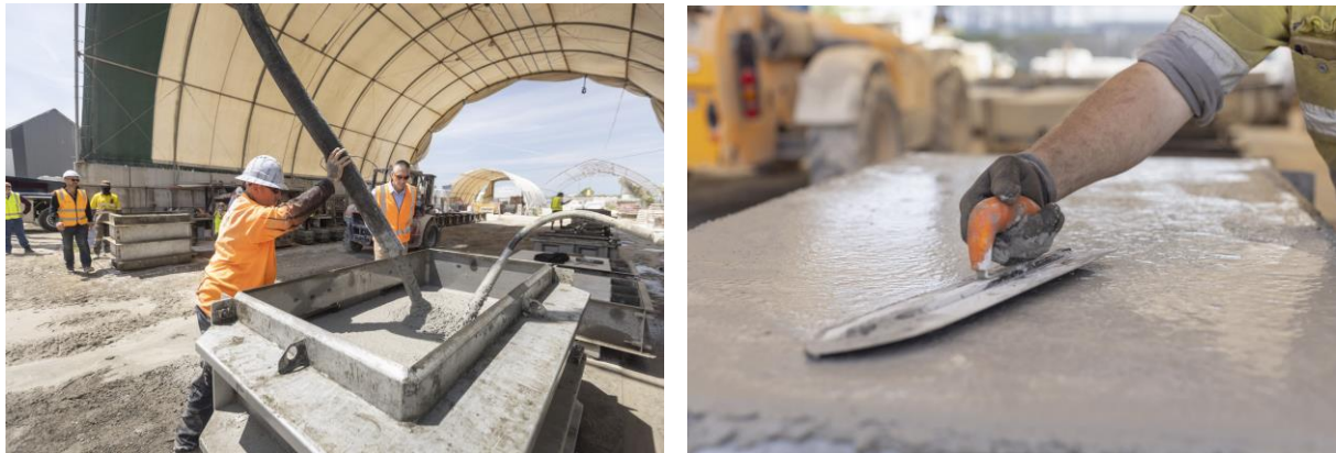
Figure 3 & 4: Wind farm concrete trials - 50% AusPozz™ mix design
